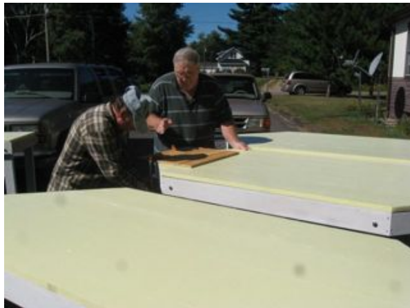
Above left, Jim and Mike are applying a bit of pressure to keep the foam glued down to the plywood as the glue sets. On the right, is a sketch of layout corner.
