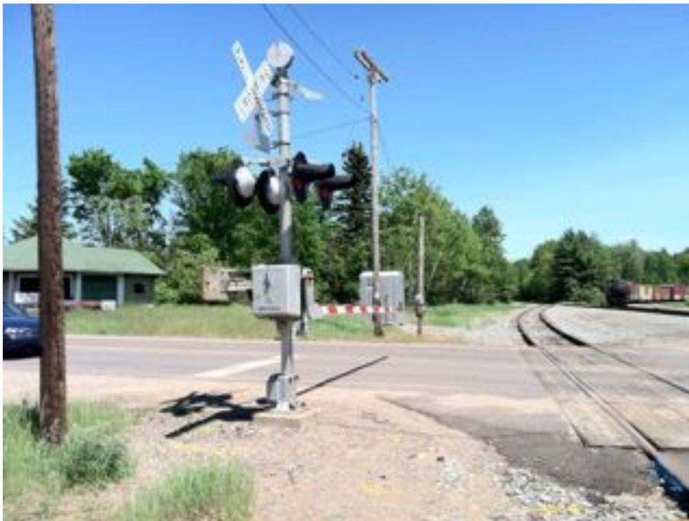
Thus, the gate operation begins with its own ringing bell at the time the engine trips the gate initiation circuit. The red flashing lights begin at about the same time. The gates then begin to slowly lower taking
