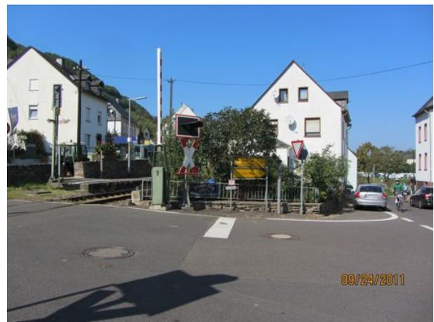
The gate crosses but one half the road; however there are two gates, both blocking the right side of the road (just like Bradley Junction on Hwy Y). Simple reflectors served to catch the motorist's eye on the gate. The warning light was mounted above the cross buck on its own post.
