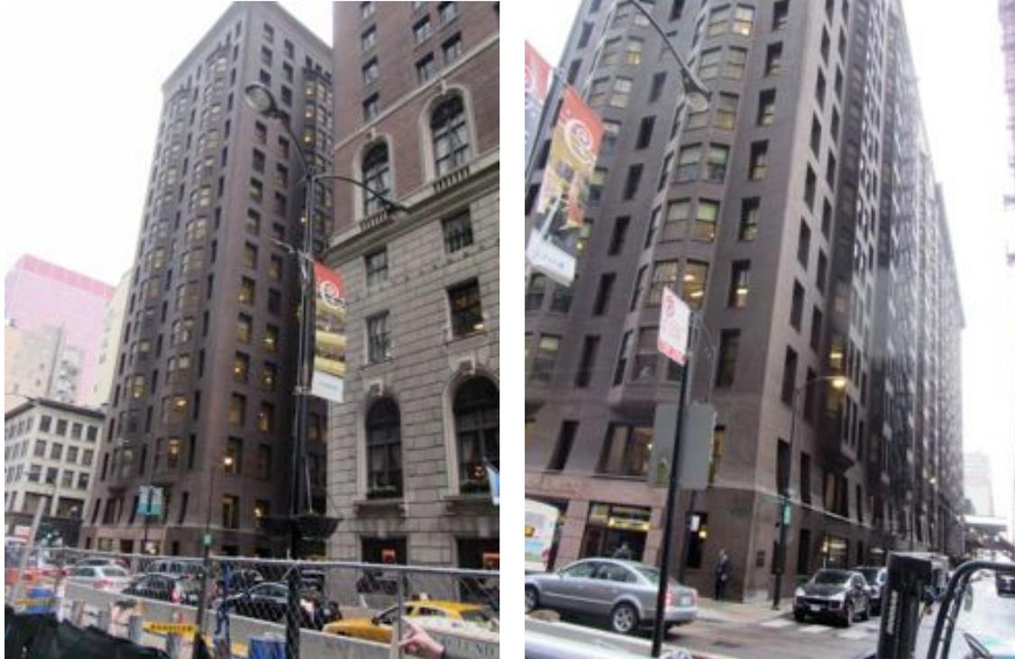
The Monadnock, when built by Burnham and Root in 1891 was the tallest building with an iron frame and exterior load bearing walls of masonry. This unusual skyscraper not only raised the population density of workers in the city; but remains the tallest building with external masonry load bearing walls in the world! Located at 53 Jackson Ave was once the largest commercial building in the world. The north half has six ft walls; south half, curtain wall.
