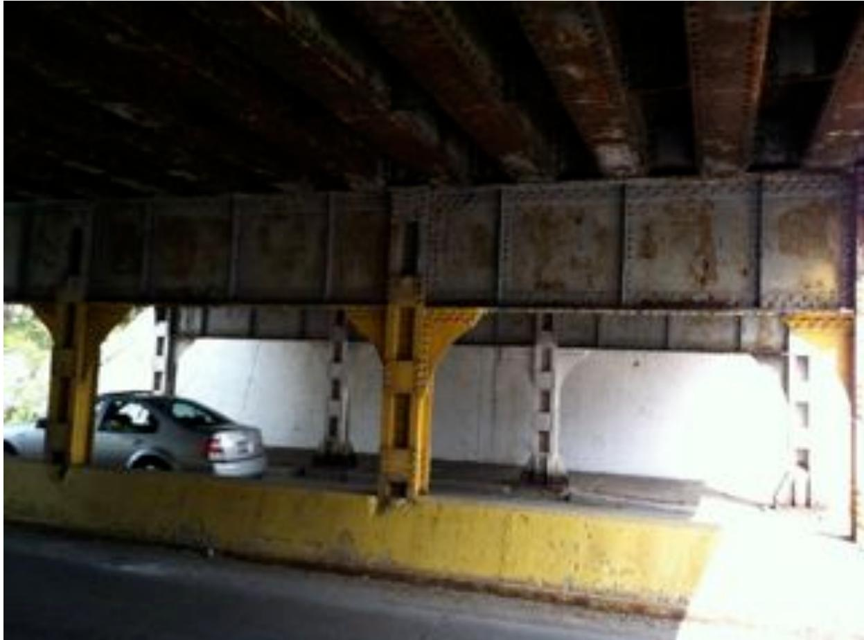
Above you find another 36 inch plate structure with 36 inch square boxes sitting on what appears to be two U flange members about 12 in wide riveted into a 12 in box frame. A concrete wall was added to keep folks from bending the bridge supports (at mid span). Five longitudinal stringers of box construction are used to support each double track main and siding above.
