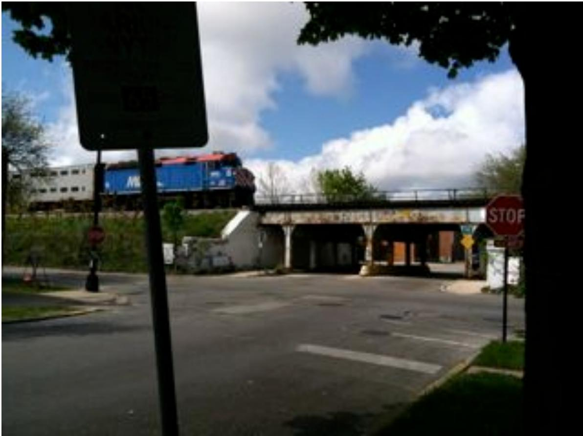
Thus the C&NW built an elevated line to remain above auto, truck and pedestrian traffic across much of the north side of Chicago and Evanston. Here at Bryn Mawr and Ravenswood we see a typical bridge and retaining wall combination. It is a bridge that is repeated scores of times in the city of Chicago and Evanston.
