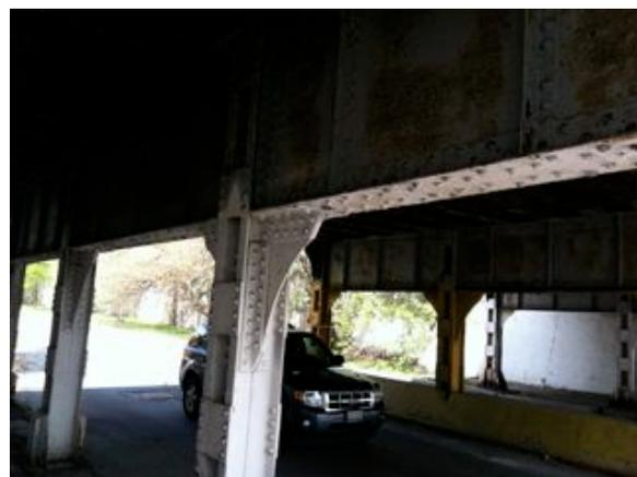
Above we see rivet and column detail. It is a highly riveted structure (that's why it has lasted). Rivets move and allow a bit of structural flex. Weldments would have been more solid, stressed, cracked and have a greater propensity for failure. Rivets while allowing movement show rust stains and paint distress (flaking, peeling and loss) at locations of movement. Hence, you can visualize how a structure is behaving by examination of its individual components.
