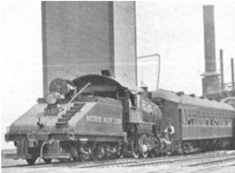
The slope back switch engine tender gave the yard crew improved visibility to the rear. It lessened the water carrying capacity; however, the yard engine was generally close to water all day long.
