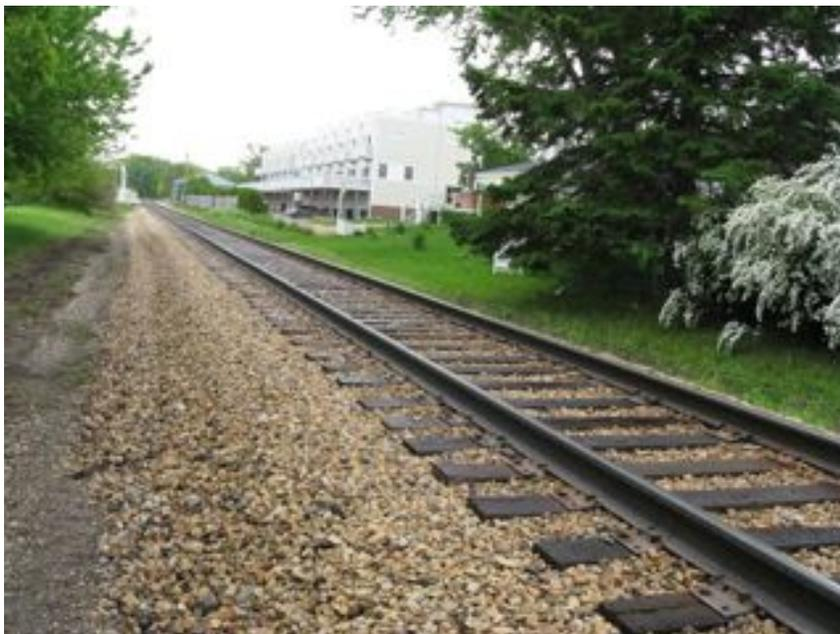
The concept of railroad ballast has much to do with tie support and drainage of water from contact with ties. On the support side of the equation we find that ties hold the track in place vertically and horizontally. To that end the ties must be trapped in somewhat an inflexible but elastic membrane of stone. Crushed stone is typically used for the purpose. The angular faces of modest size stones lock the tie in position while being porous and allowing drainage.
